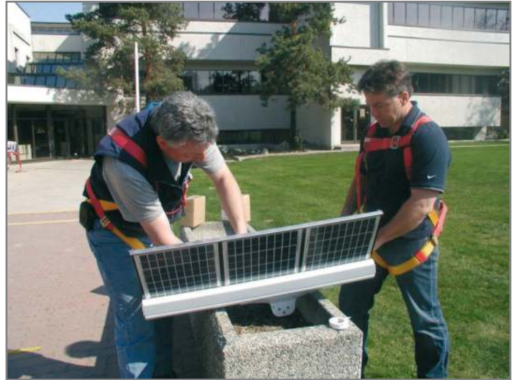
Figure 3: Preparation of the solar engine for installation at the pole by qualified personnel
