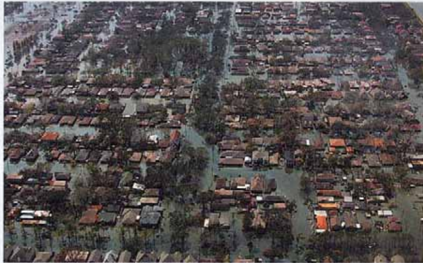
With PV back up systems, operation of crucial infrastructure could have been continued in flooded New Orleans. But the Gulf Coast states hit by Katrina offer hardly incentives.
