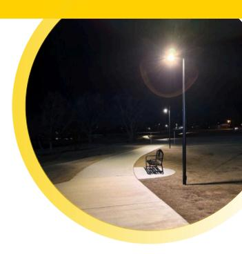
Fifteen UP2 units now illuminate the completed sections of the trail. Installation was fast and straightforward: poles were direct-buried into the ground, with no need for concrete footings. On phase two added expanding foam for peace of mind, but it's been a smooth process."
